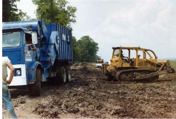
Unit 10: Operations and General Health and Welfare
